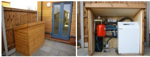
Figure 3.12 Heat pump external housing and contents
